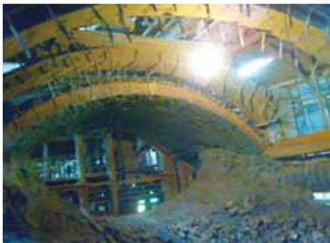
Fig 3 Twin hearth furnace roof during dismantling
